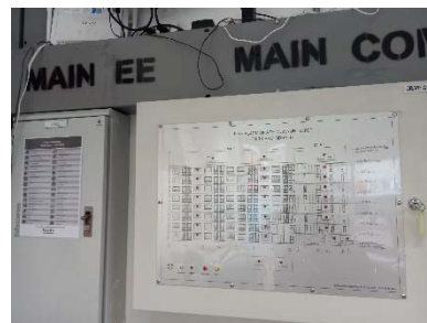
Graphic Annunciator Fire Alarm System
